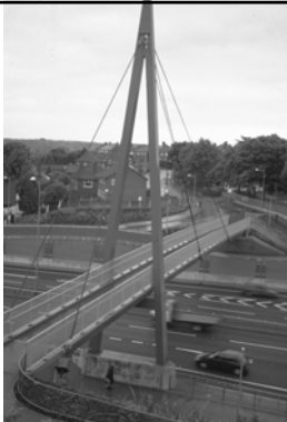
Box Lane Footbridge
