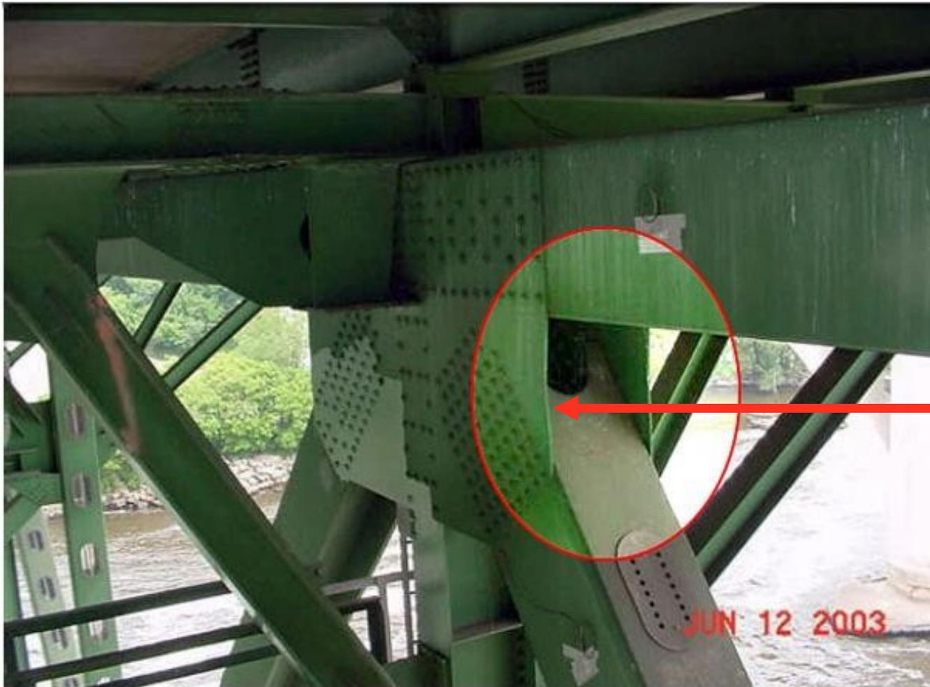
This photo from June 12, 2003, shows a bent gusset plate on the I-35W bridge that is visible to the eye. (Photo courtesy of NTSB)
