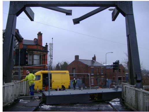
After failure with counterweight across carriageway
