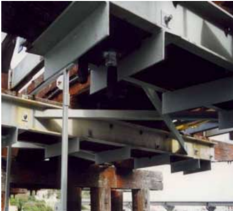
Figure 8: Transom Beam Strengthening
