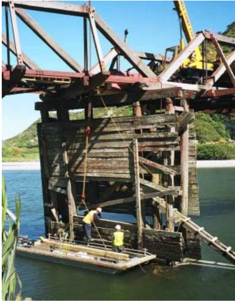
Figure 3: Typical Pier Detail & Transom Beams
