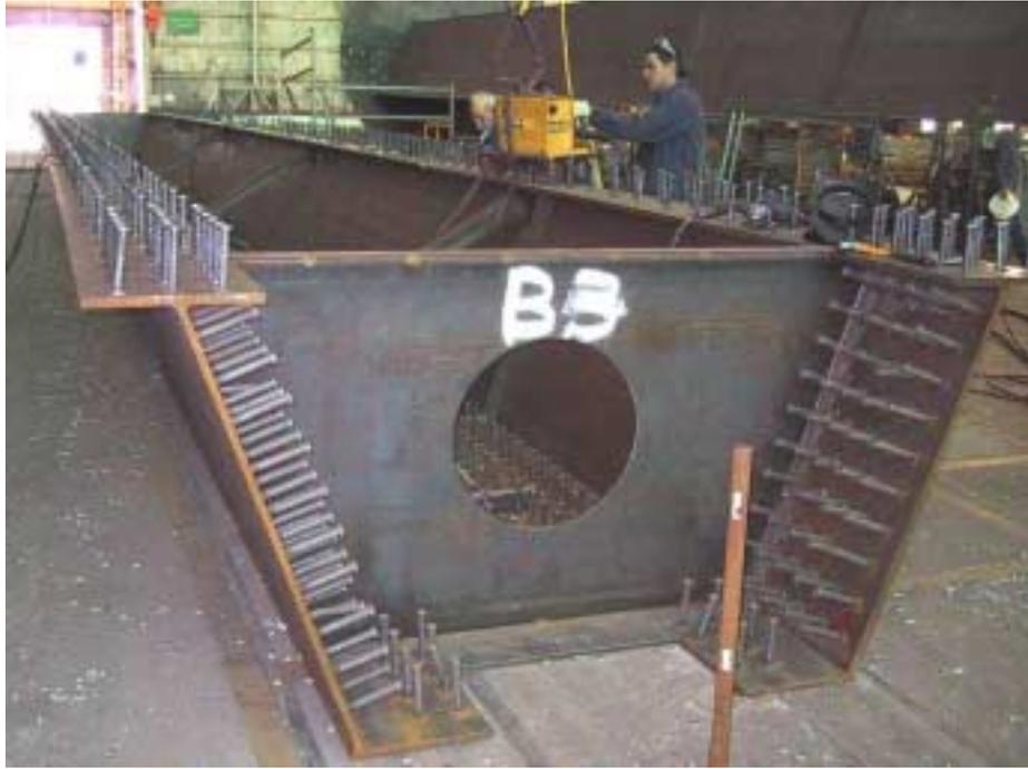
*Figure 4: Typical Box Girder under construction*
