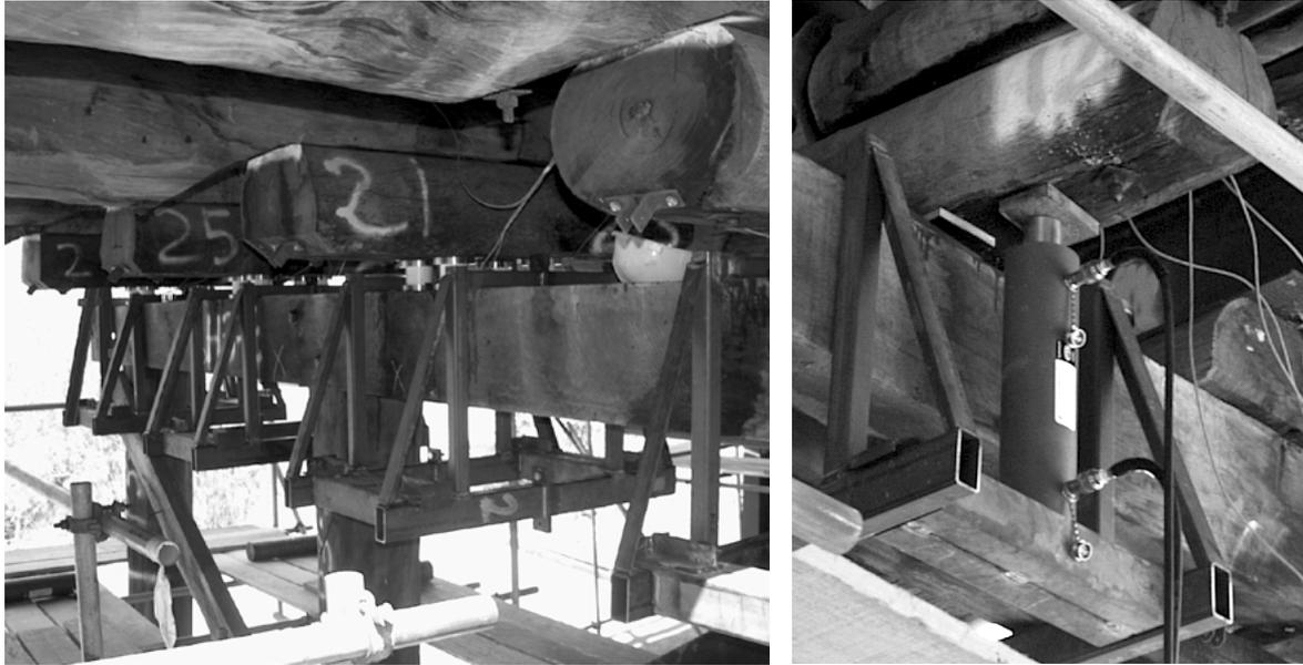
***Figure 3: Purpose-Built Frames Used To Lift the Bridge Superstructure To Insert Loadcells***
