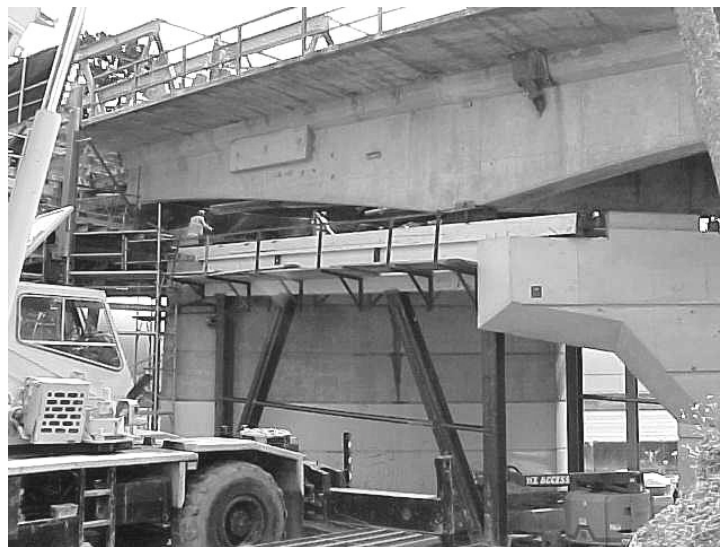
Photo 2: Bridge Sliding Showing Runway Beam
