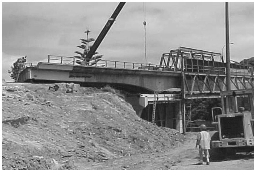
Photo 3: Bridge Sliding Showing Temporary Decking
