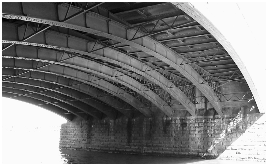
Figure 3 Underside of Princes Bridge
