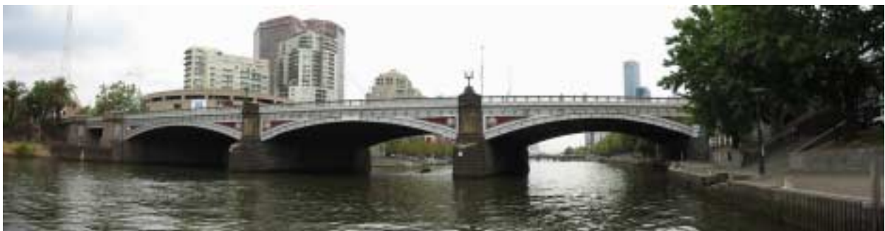
Figure 1: Princes Bridge, St Kilda Road, Melbourne, Australia
