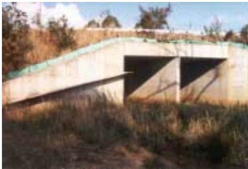
Fig.12: Fauna underpass with natural base cover and an elevated lizard run for reptiles and small terrestrial fauna.
