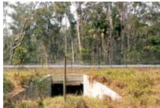
Fig. 14: Typical fauna underpass with refuge pole at entrance. Clear sight through culvert encourages use.
