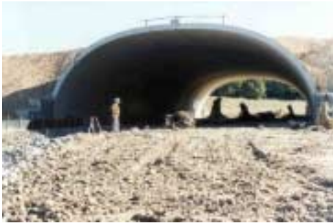
Fig. 11: Large buried arch type fauna underpass. In this case the span exceeds 20 m, which is more than double the required dimension.
