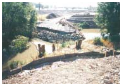
Fig. 4: Good control on water pollution - temporary rock platform for pier constructed in watercourse.
