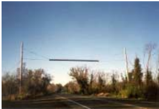
Fig. 15: Suspended fauna funnel – suitable for possums.
