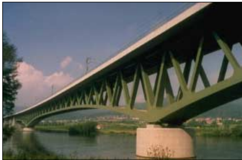
Figure 5: Dual composite Railway Bridge across the Main River, Germany
