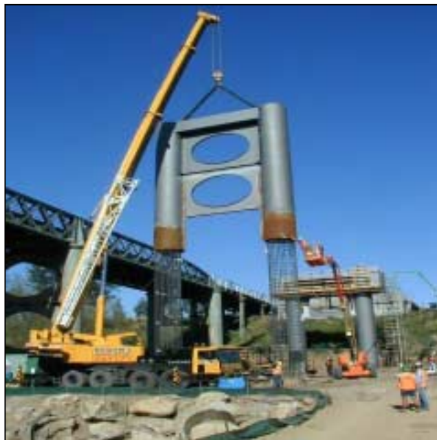
Figure 8: Under Construction: Erection of Pier 18
