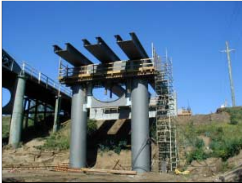
Figure 6: Under Construction: Trough Girders erected
