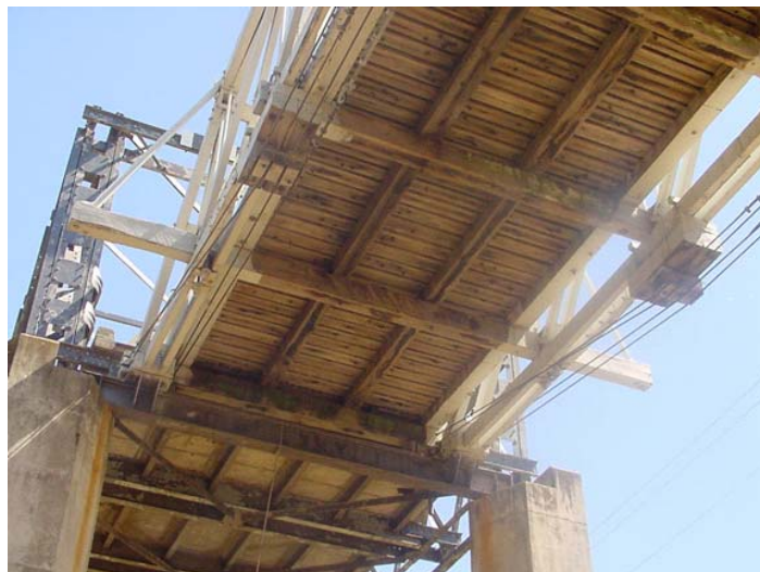
Figure 1. Heritage Truss Bridge (including cross-girders) Typical of RTA Structures
