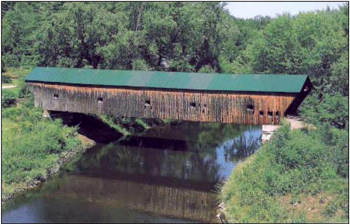
Figure 4: Hammond Bridge, Vermont (Town lattice truss, 1842)
