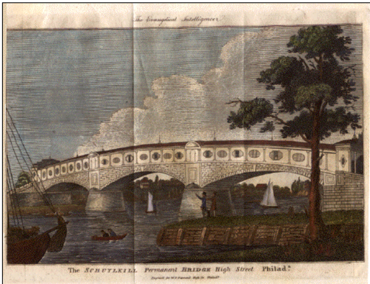
Figure 3: Schuylkill River Bridge, Philadelphia, Pennsylvania (1805)
