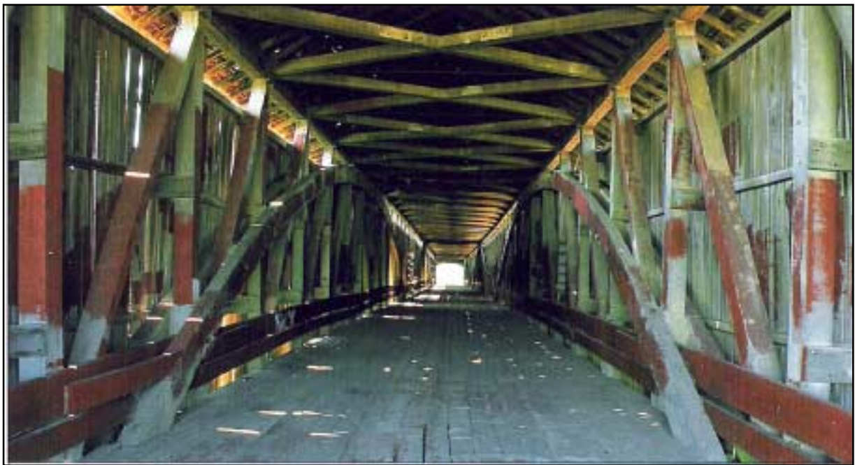
Figure 5: Medora Bridge, Indiana (Burr arch/truss, 1875)
