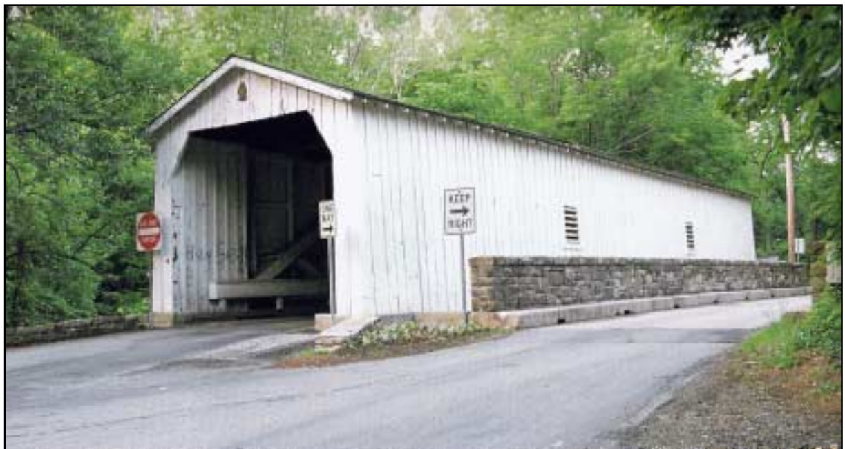
Figure 7: Green Sergeants Bridge, New Jersey (Queen truss, 1866)
