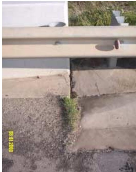
***Figure 13: View Showing Gap of Less Than 10mm at End of Abutment***
