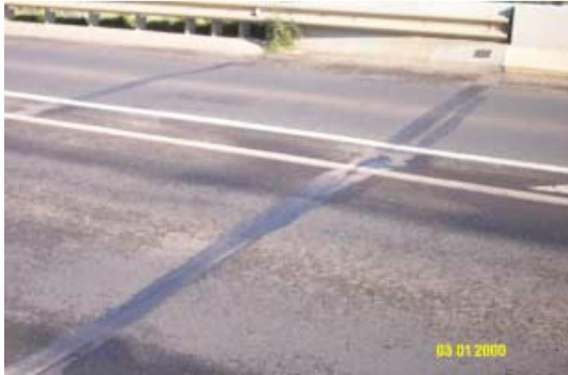
**Figure 14: Approach Pavement Crack and Joint Filling**
