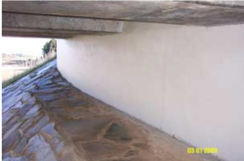
***Figure 12: Front of Abutment Showing Condition of Rock Beaching***
