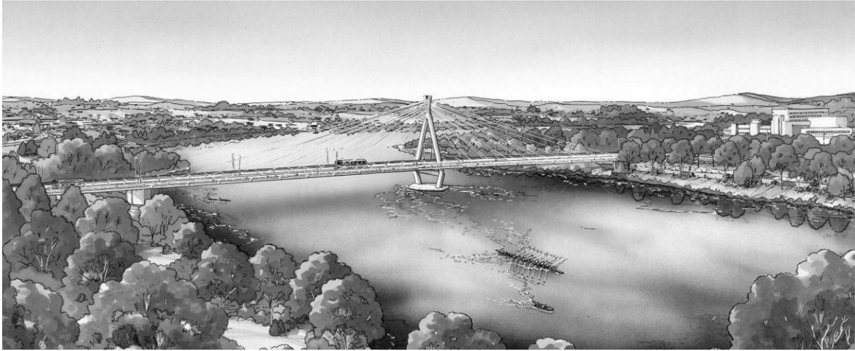
*Figure 4: Option 3 - Single tower cable stayed bridge*
