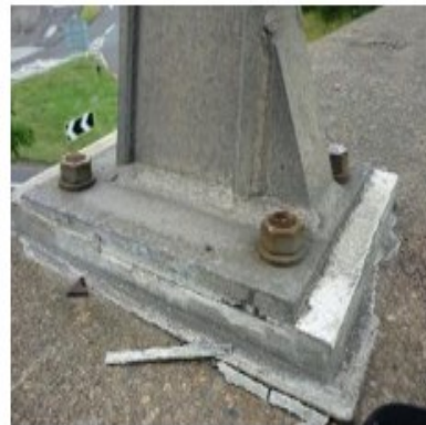
Post-installed parapet fixing
