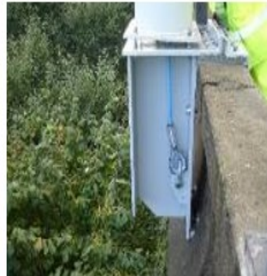
Gantry attached to bridge parapet
