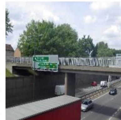
Sign fixed to bridge
