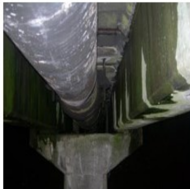
Utility suspended from bridge deck
