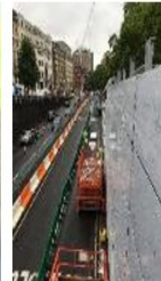
Cladding system in underpass
