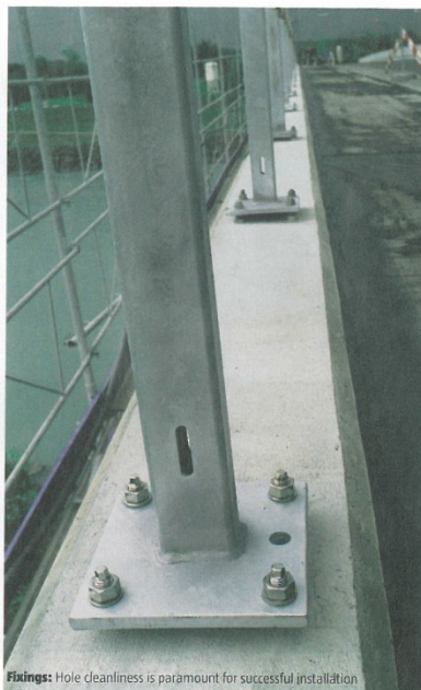
Fixings: Hole cleanliness is paramount for successful installation
